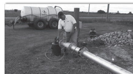
View of fertigation system with check valves and portable tank.
